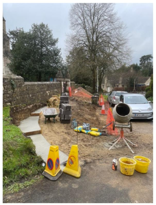
✓ A more accurate arc was plotted on the new concrete foundations to form the building line for a double wall comprising concrete blocks at the back and solid dressed stone for the facing.
