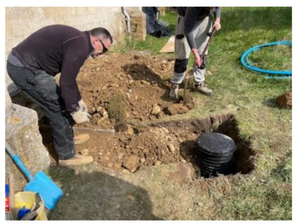
✓ The associated pipes and bends from the back of the toilet and basins was arranged in the corner of the toilet area. Type 1 (gravel) was tipped in the hole with some of the original spoil to a level 100mm below finished inside floor level. Limecrete will be laid to bring the final level up to 25mm below floor level to enable the floor tiles to be relocated.
