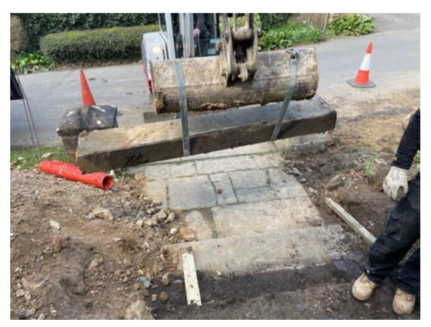
✓ Using a laser, the levels for the ramp were set out prior to construction work. The radius for the ramp was marked out taking into consideration the low walls on each side of the path. At this point, whilst driving in a peg to support the shuttering, Will
