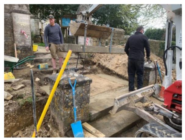
The two lower steps were fixed in place and the restraining concrete block walls were constructed before laying the upper treads.
