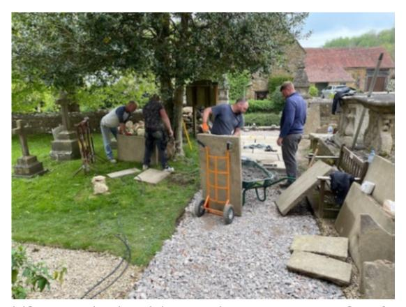
While Jon mixed and barrowed a constant supply of mortar, the slabs were set down, carefully followed by Doug who grouted the joints between each stone.
