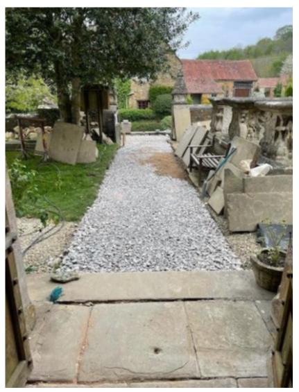
Jon and Doug barrowed Type 1 stone chippings from a delivery by the roadside and laid to form a slight gradient up to the porch threshold. A laser was used to confirm the incline angle. The gravel was finally compressed with a vibrating plate before the slabs will be relaid next week.
