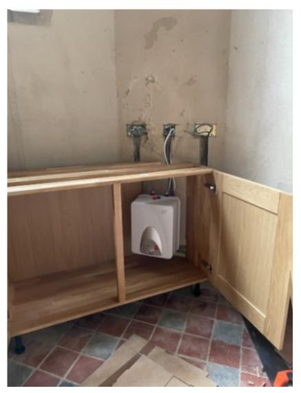
✓ The pipework for the cold water supply to the heater and kitchen sink taps was fitted with all the associated joints and bends. The hot supply and waste was also attached to the wall and fed through to the area behind the toilet. Simultaneously, the water supply and waste to the hand basin in the toilet were fitted. Final wooden linings were fitted to the openings behind the toilet in readiness for plastering.
