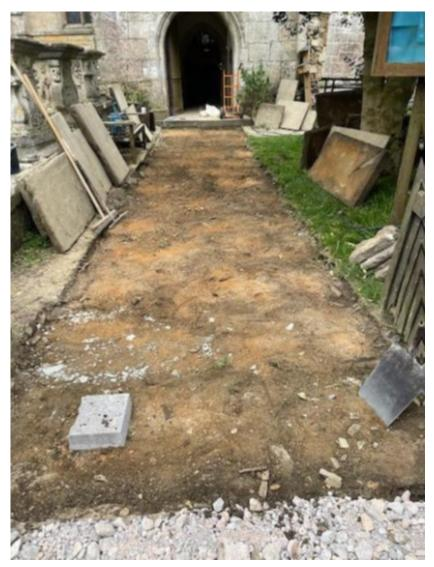
Jon and Doug carefully lifted each stone slab, marked them with a letter and a plan made of their positions so that they could be re-laid in exactly the same order.
