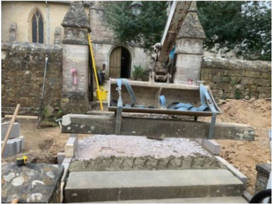
By the end of the week all five treads had been replaced. The original steps had slightly sunk over time such that they were tilting backwards. This had the unfortunate result of holding any rainfall at the back of the treads. Having now repositioned the steps correctly has consequently increased
