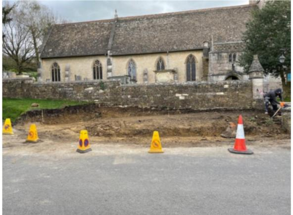
✓ Shuttering was set up to form a framework into which concrete will later be poured for the foundations of the low walls. More concrete will be poured behind the low walls to underpin the existing stone wall above. The existing
