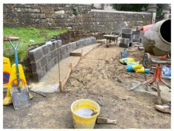
✓ A row of concrete blocks were laid on the curve on top of the concrete that will serve to hold back the earth between the new wall and the existing church boundary wall. More concrete will be poured into the gap after the concrete blocks have cured
